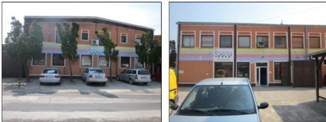
Figures 1 and 2: Office space - Directorate - Street and yard views
