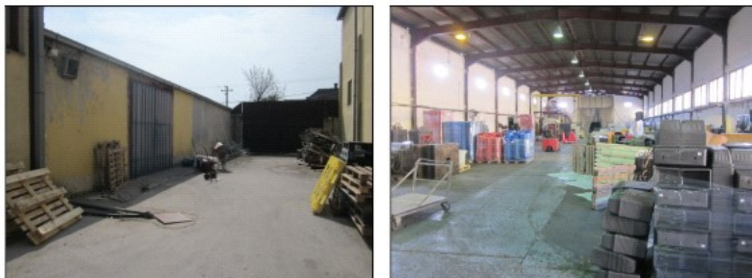
Figures 3 and 4: Production hall with workshop - yard view and interior
